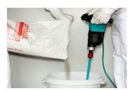
Prepare Floor Leveling Compound C15 3116 or Floor Leveling Compound FX 3109 without lumps using a suitable mixer (e.g. Collomix Xo 4 R HF 3347) and stirring rod.
