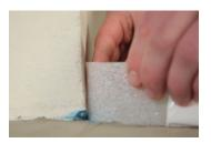
Vacuum and clean prepared floor surfaces. Install Perimeter Insulation Strips SK 3018. Check compatibility and adhesion to the substrate, especially for finished surfaces, in advance by conducting a sample bond.
