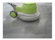
For the further build-up, sand the smoothly filled surfaces in advance using a single-disc grinder (grit size P60 / P80 as a cleaning step) and vacuum. Also clean and vacuum the edge insulation strip of any residual leveling compound.
