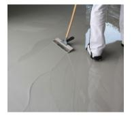
Then texture and design individually using the Surface Filler Knife 1828 with Handle Socket. It is best to work diagonally or in a diagonal direction. Do not level at right-angles or linearly. The size and type of the tool determines the character of the texture. The smaller the tool, the more concise the texture pattern.
