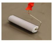
Work through the fresh leveling layer with the de-aerating roller in a criss-cross pattern
